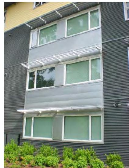
increase ventilation rates. When design permits, provide windows in stairways and corridors to introduce natural lighting. Consider children's safety when choosing how the windows will open and close. Confirm the type of window coverings with the operator. In determining whether windows should open, consider ventilation needs and consult with the operator about program needs. Some security systems prevent windows from being opened.
